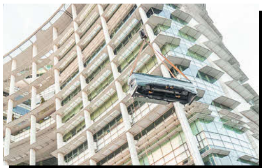
↑ Major works to replace chillers with more energy efficient models
