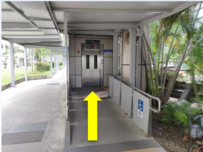
5. Enter the lift and head to the other end of the overhead bridge
